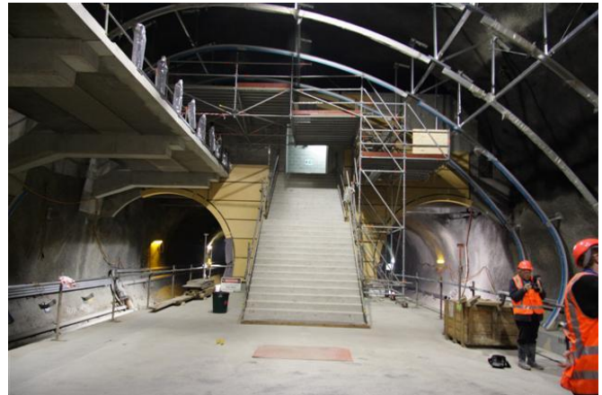
Figure 2: Using of NATM method for station construction
