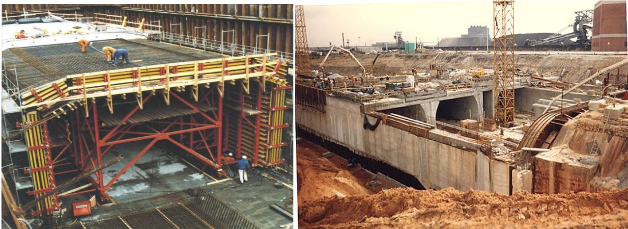
Fig. 4: Cut and cover construction method
