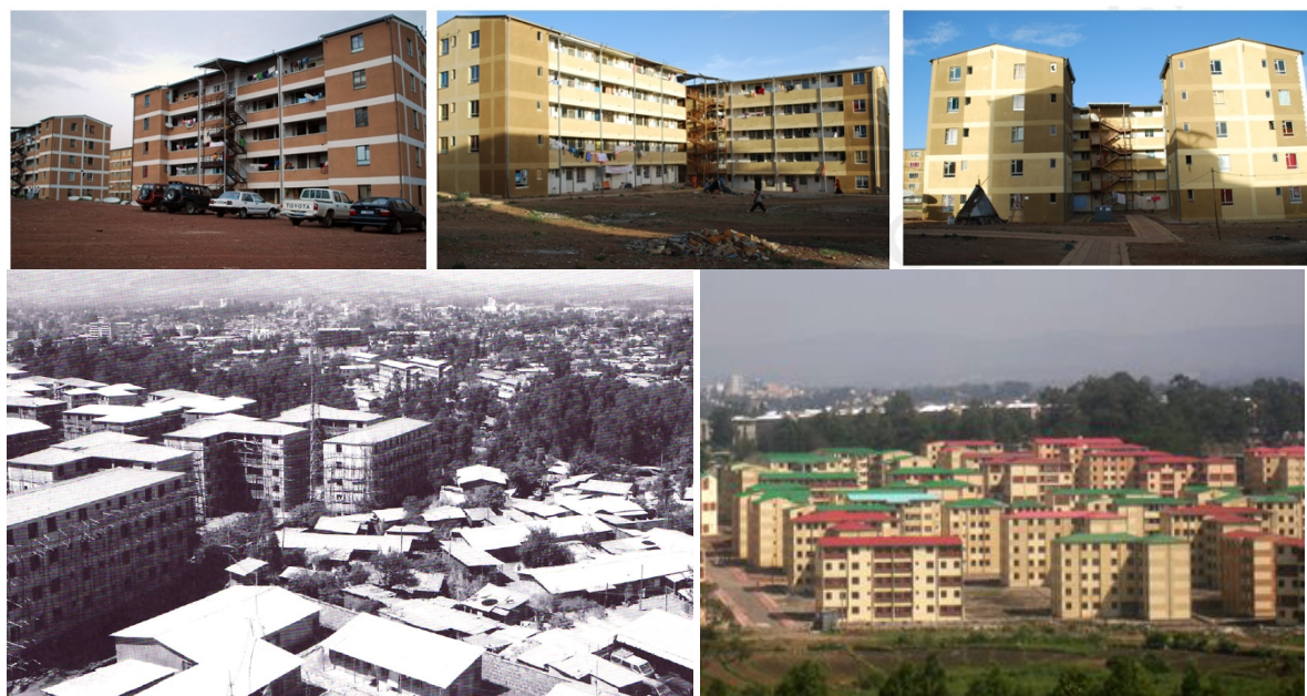
Figure 12-16. The popular condominium blocks Type-C and block Types B and D (from left to right). (a) New condominium next to existing neighborhood; Source: Angelil & Hebel 2009 (b) cluster of condominium blocks at a suburb in Addis.
